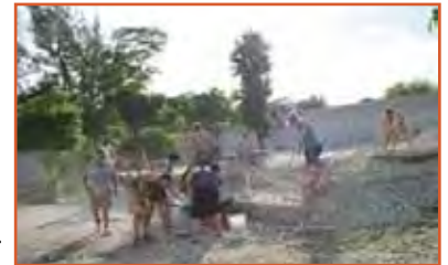
Team working hard on slab demolition
