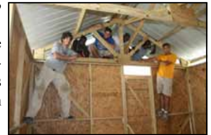
Working on the Bungalows
