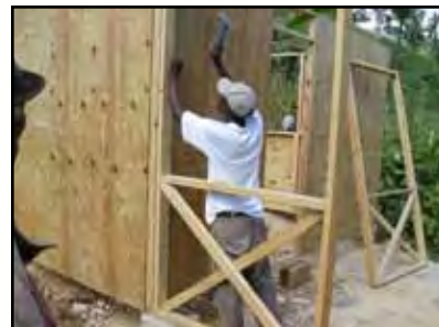
Adding the Porch
