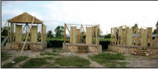
New homes being constructed on their hurricane resistant foundations.
