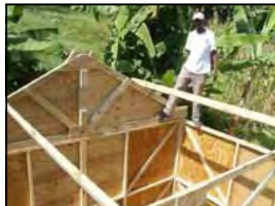
Bulding the Rafters
