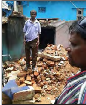
Mark's Collapsed House
