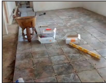
Tile on our floor is nearly done
