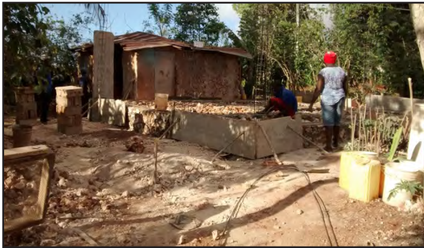
New foundation with old home in back
