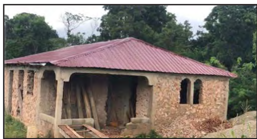
Jean Fouca's New Roof
