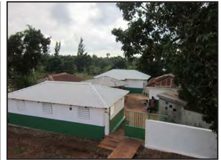
The hospitalization center with improvements
