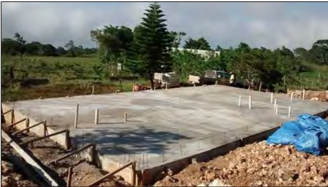
Foundation for our house
