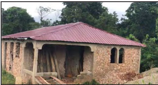
Jean Fouca's New Roof
