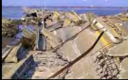
Used to be a Highway
