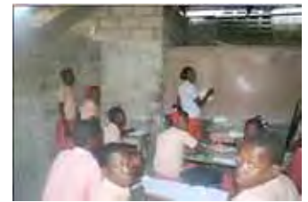
All the classrooms need major repairs
